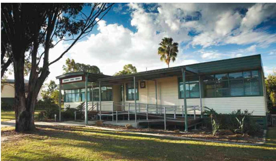
Top: The partnership will provide new opportunities for trade training. Above: Wandoan State School
